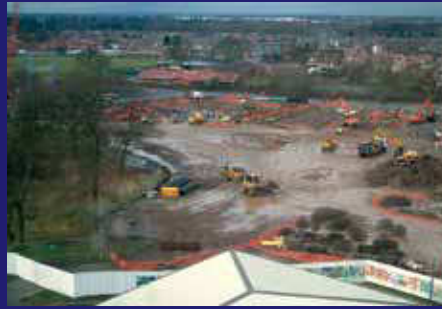
January 2009 - The drainage systems on the new site are installed.
