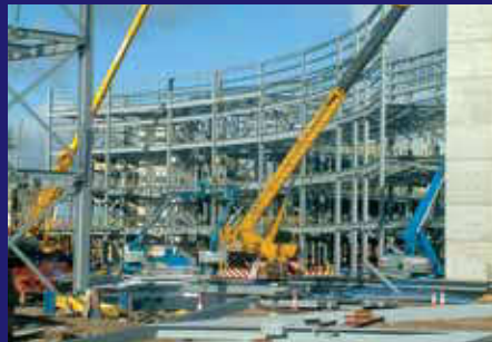
April 2009 – Steelwork continues to rise.
