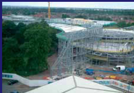
June 2009 – Steelwork continues to progress well.
