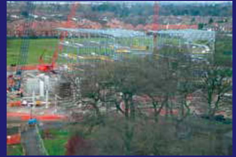
February 2009 – The new steelwork takes shape.
