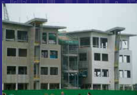
July 2009 - The concrete framed library rises up.
